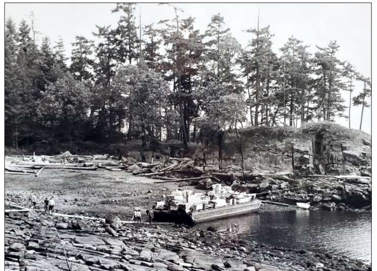
The barge in position Number Two
